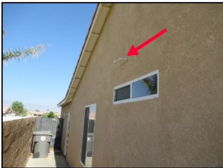
A/C condensate lines - recommend re-positioning away from house Image showing A/C drain line routed upwards, not allowing water to drain properly
